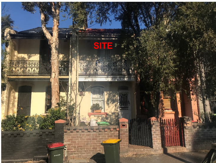
Figure 2: Site viewed from Charles Street
