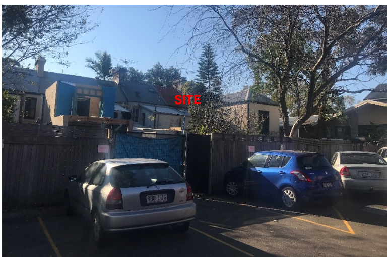
Figure 5: Viewed from carpark adjoining to the rear
